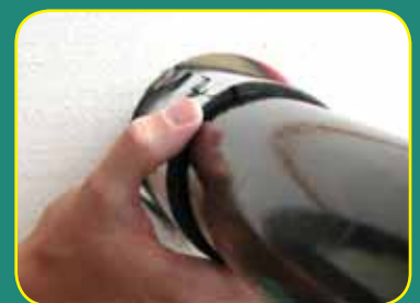
2: Placing Fire Sleeve
